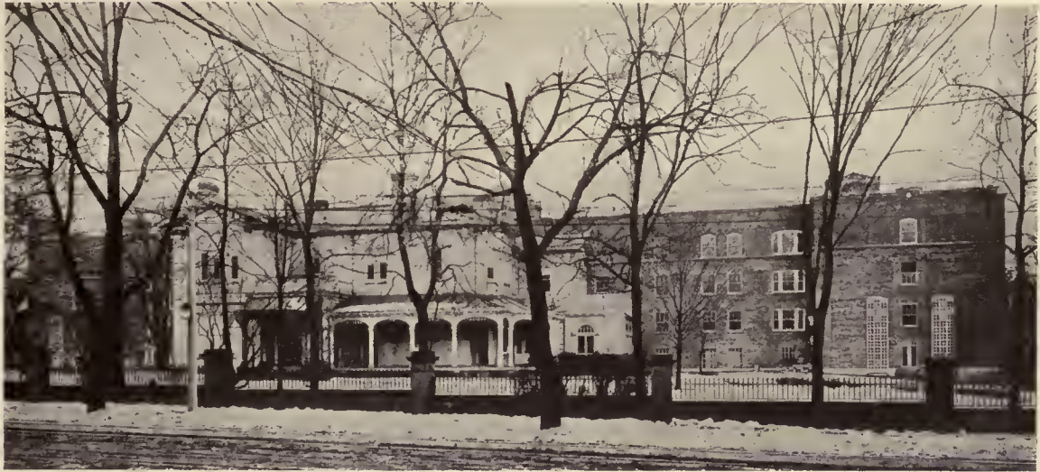
SHERBOURNE HOUSE CLUB ROBERT SIMPSON COMPANY, LTD., TORONTO, CANADA N. MAX DUNNING, ARCHITECT
